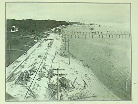
MISSISSIPPI GULF COAST Concrete paving and curved sea wall protection at Biloxi costing \$100,000 per mi. 29 mi. of sea wall, paving and concrete bridges now nearing completion. The sea wall now building is a different type. 22
