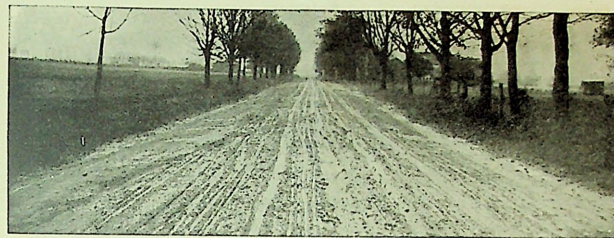
HIGHWAY TWO DAYS AFTER COMPLETION
