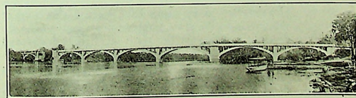
Section of Apalachicola River Bridge, Florida, during construction. Total length 5500 ft.
